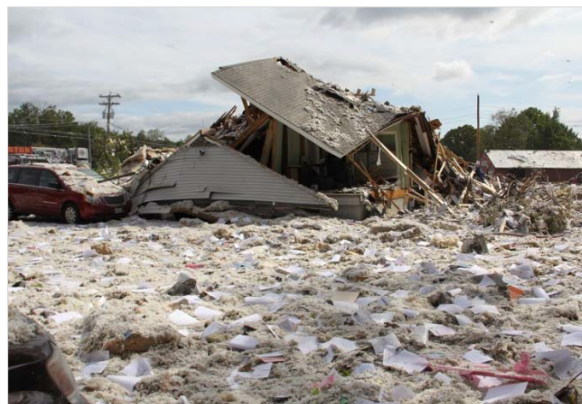
Debris field from the propane explosion described in the FFFIPP Investigation
