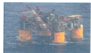
NCP/NRS Response: Oil discharge from a damaged offshore facility following an accident. RP can be identified and the Federal On-Scene Coordinator will respond under NCP authorities and funding mechanisms.
