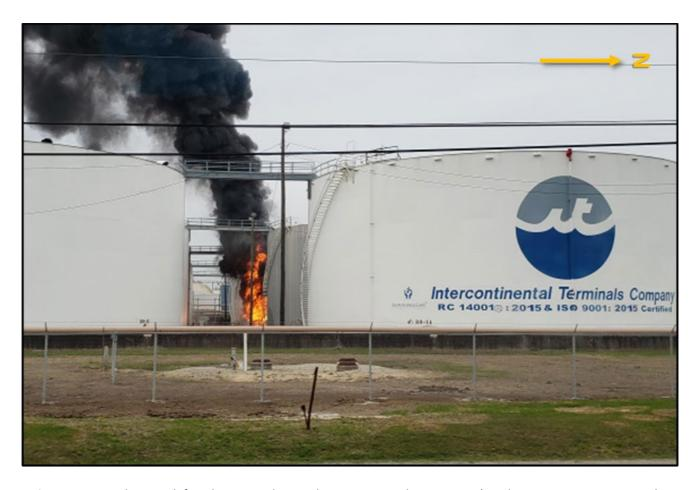
**Figure 11.** Initial ITC tank fire that ignited at Tank 80-8 on March 17, 2019. (Credit: HCFMO, annotations by CSB)
