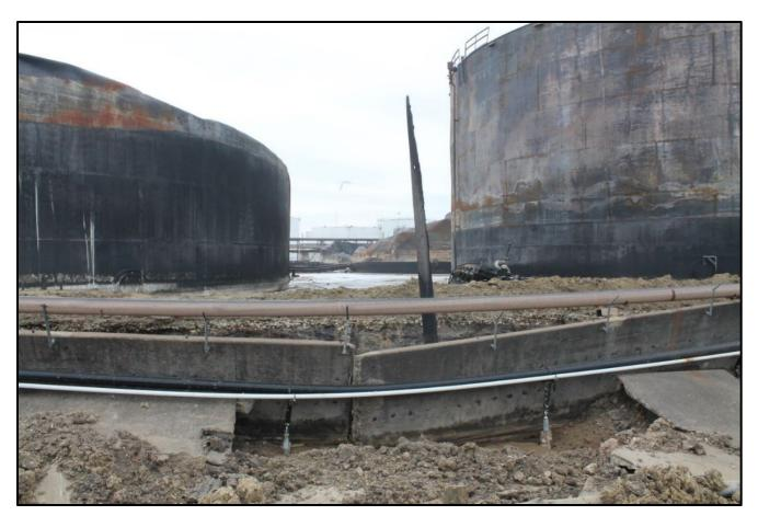
**Figure 17.** Close-up view of the First & Second 80's tank farm containment wall breach that occurred on Friday, March 22, 2019. (Credit: HCFMO).
