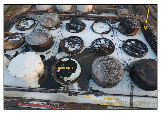
**Figure 16.** Overhead view of the First & Second 80's tank farm containment wall failure that allowed materials to enter the surrounding waterways on Friday, March 22, 2019. (Credit: ITC, annotations by CSB)
